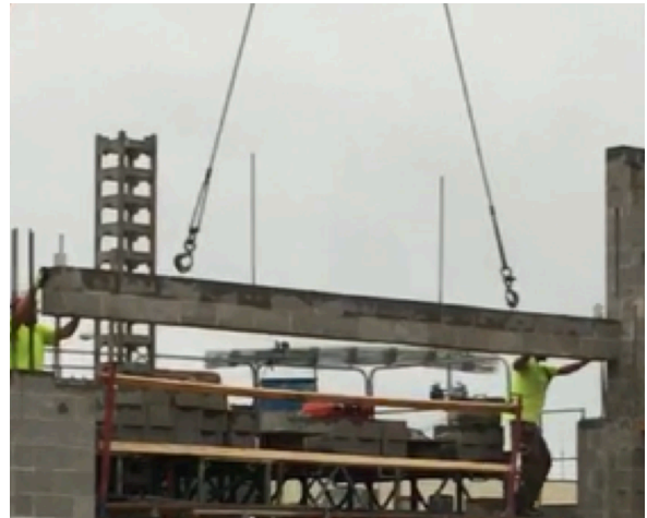
Figure 1: Prefabricated Masonry Lintel
